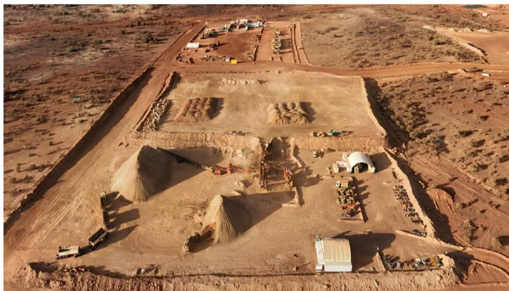
Figure 2.4 - Crown Prince ROM & Crusher Pad
