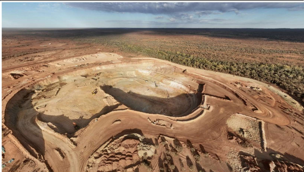
Figure 2.3 - Progression of Stage 1 Pit Inside Larger Stage 2 Pit Boundary
