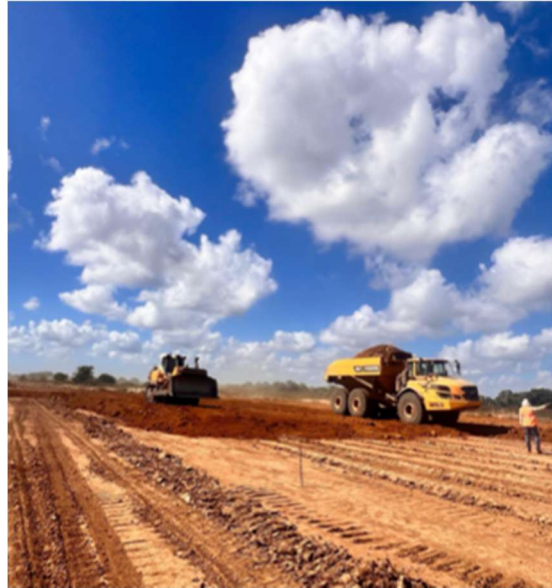
Figure 3.2 – Construction underway at Nueva Sabana
