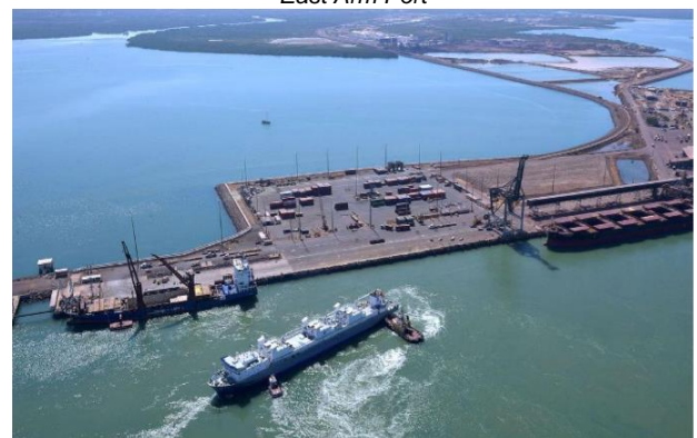
Berth 2 bulk berth (ship docked)
